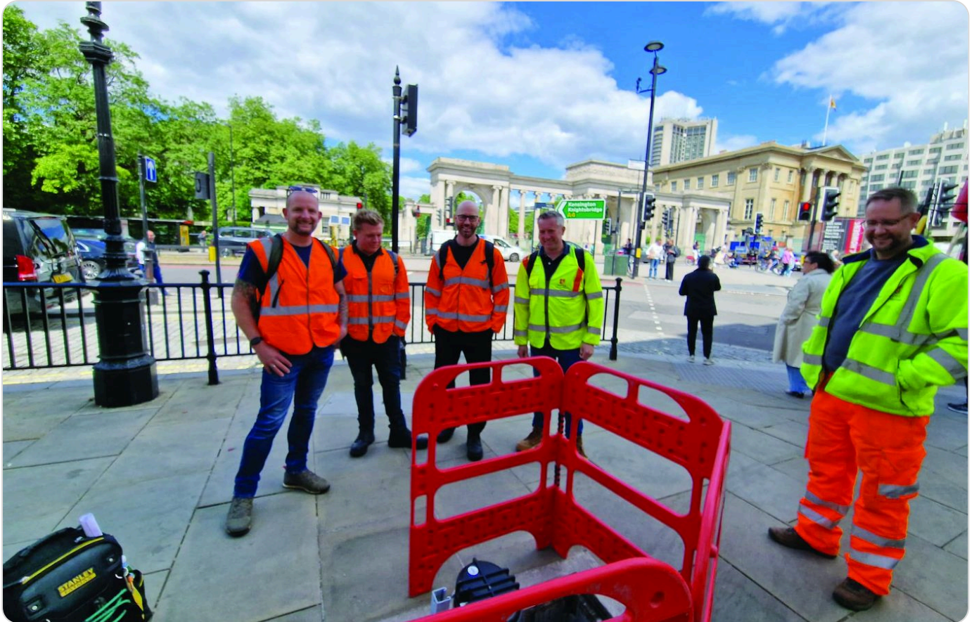
STREETWORKS IN CENTRAL LONDON. BOLDYN BUILD PARTNERS ON SITE
